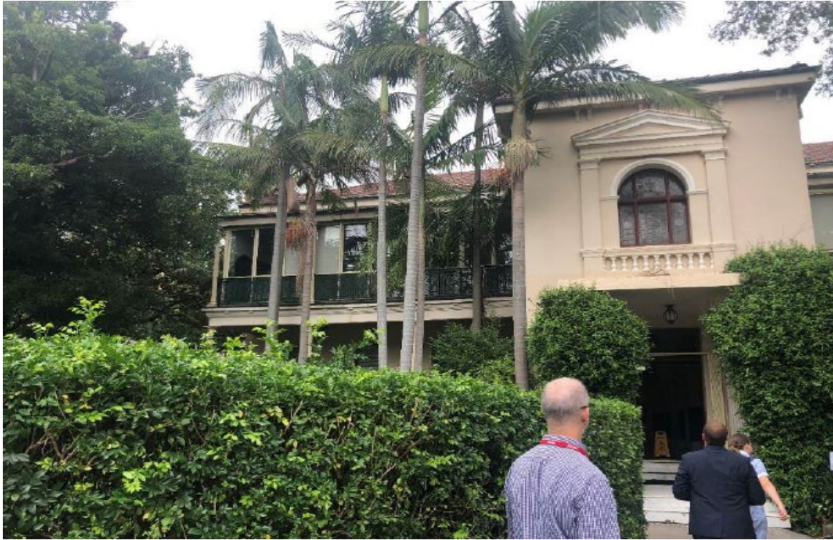
east elevation of Administration Building
