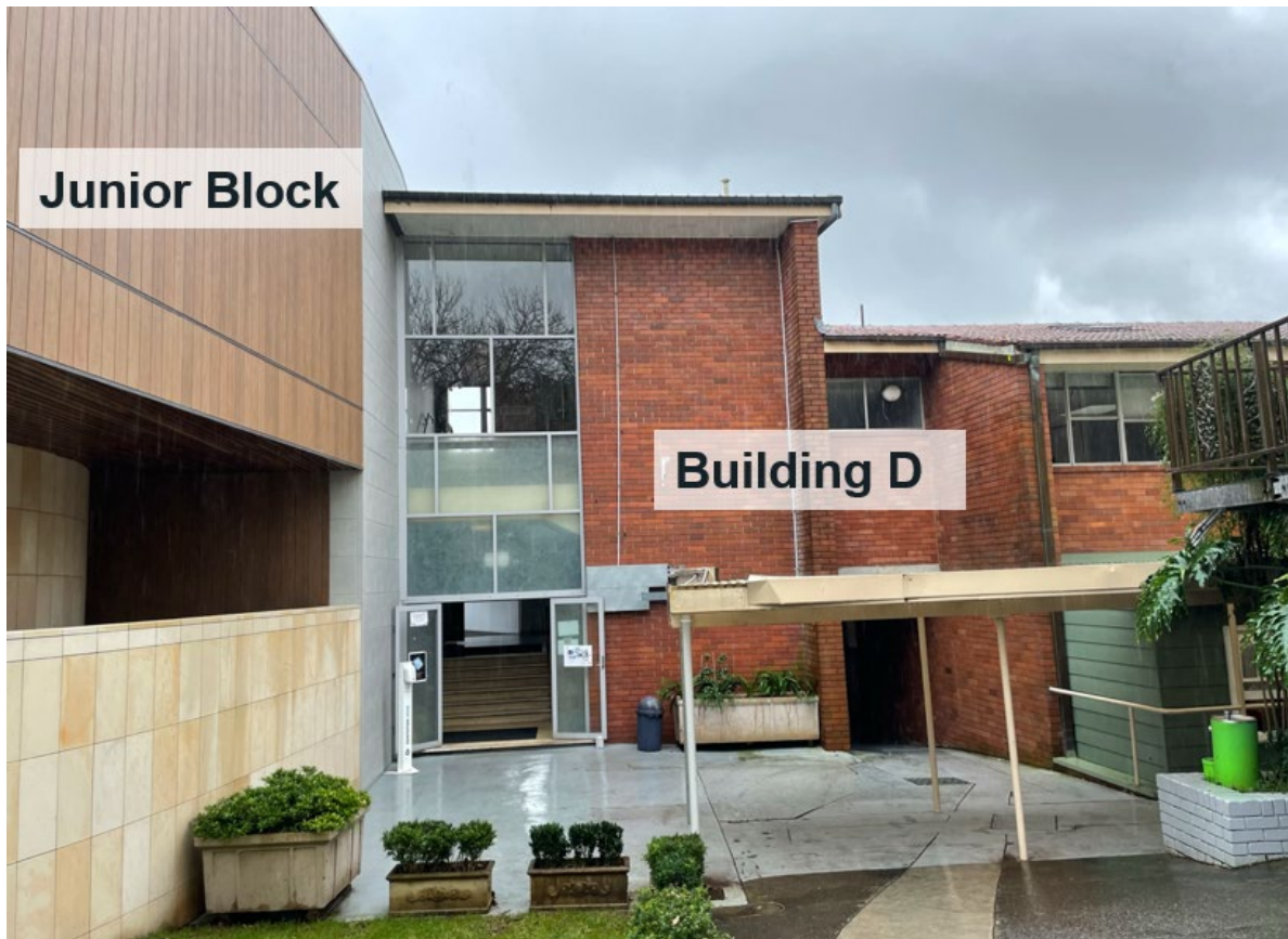
east elevation of the Junior Block and Building D
