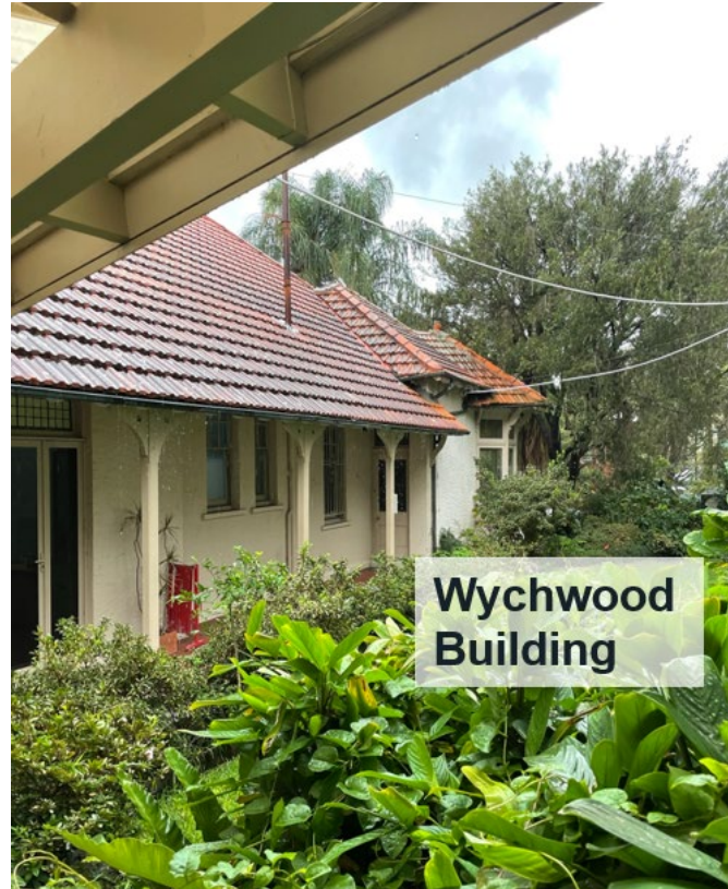
South elevation of Wych Wood Building
